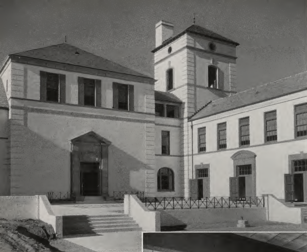
One of many beautiful, firesafe concrete masonry schools in California is the Beverly Hills High School. The concrete tile exterior was given a light stucco wash. Designed by Robert D. Farquhar and built by Henry W. Schlueter.
